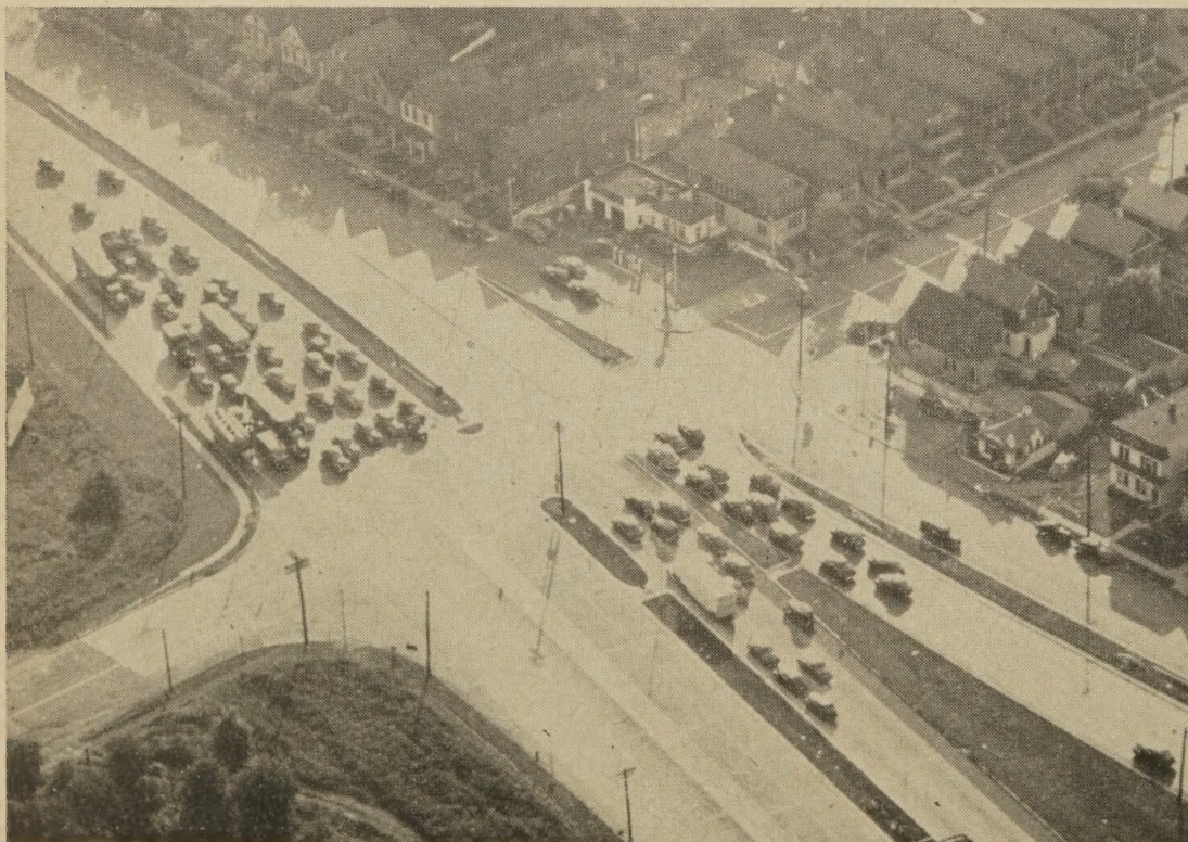
An intersection on a high-type facility. The traffic volume is near the practical capacity of the intersection, although between intersections the highway is adequate for a much greater volume.
